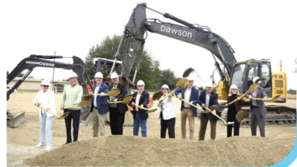
Groundbreaking of the Skagit County Crisis Stabilization Center
